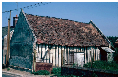
Grange. Phot. Martine Plouvier IVR22_19836000339ZA
