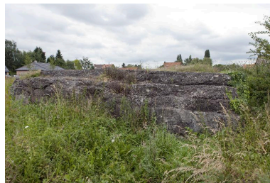
Casemate à personnel (Bat. B) Phot. Jean-Marc Ramette IVR31_20145904720NUCA
