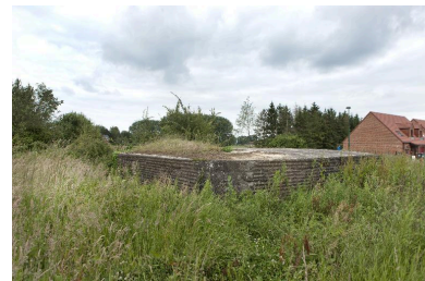
Casemate à personnel (Bat. B) Phot. Jean-Marc Ramette IVR31_20145904719NUCA
