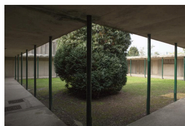
Cloître. Phot. Pierre Thibaut IVR31_20155900180NUCA
