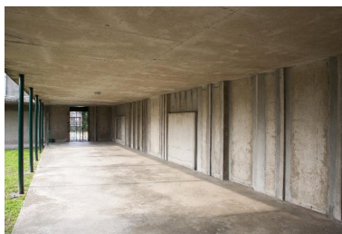
Cloître. Phot. Pierre Thibaut IVR31_20155900183NUCA
