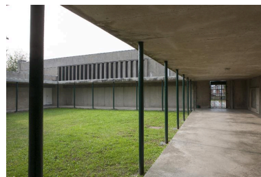
Cloître. Phot. Pierre Thibaut IVR31_20155900182NUCA
