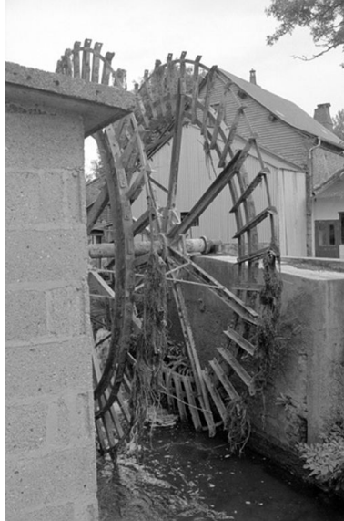
Roue hydraulique. Phot. Francis Dubuc IVR22_19908000604Z
