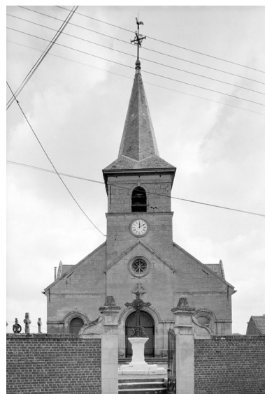
Façade occidentale. Phot. Jean-Michel Perrin IVR22_19846000961X
