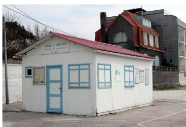
La station de sauvetage. Phot. Elisabeth Justome IVR22_20058003749NUCA
