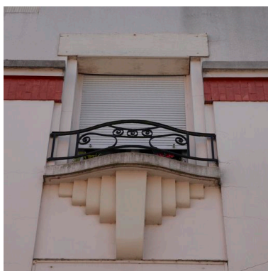
Appui de baie pyramidal. Phot. Pierre Thibaut IVR31_20096200206NUCA
