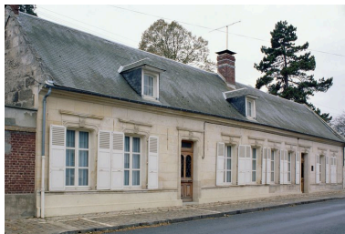
Elévation antérieure. Phot. Alain Nafilyan IVR22_19856001458ZA
