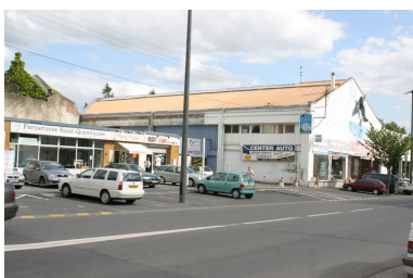
Atelier, boulevard Henri-Martin. Phot. Frédéric Pillet IVR22_20050206055NUCA
