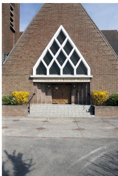
Porche. Phot. Pierre Thibaut IVR31_20155900927NUCA
