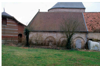
La chapelle. Phot. Irwin Leullier IVR22_20008000118ZA
