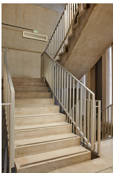
Escalier est. Phot. Pierre Thibaut IVR22_20225900484NUCA
