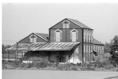
Atelier principal, flanc sud-est. Phot. Francis Dubuc IVR22_19908001252Z
