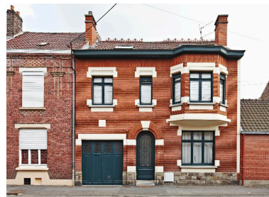
Maison, 37, rue Boeynaems. Phot. Hubert Bouvet IVR31_20105900141NUCA
