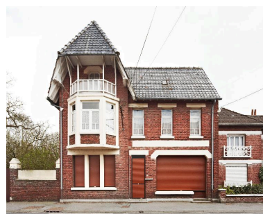
Maison, 23, rue Boeynaems. Phot. Hubert Bouvet IVR31_20105900143NUCA
