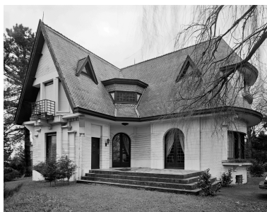
Elévation occidentale. Phot. Olivier Marlard IVR31_19935901924V
