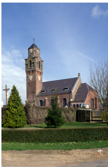
Elévation sud. Phot. Christiane Riboulleau IVR22_19960200462ZA
