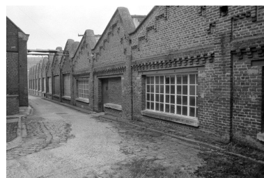
Atelier de fabrication, flanc est. Phot. Benoît Dufournier IVR22_19878000430Z
