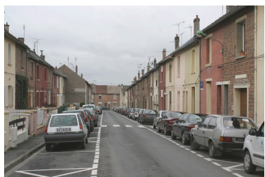
La cité Ducret, rue Albert-Daltroff. Phot. Frédéric Pillet IVR22_20060205019NUCA
