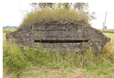
casemate h, pignon nord Phot. Jean-Marc Ramette IVR31_20145904933NUCA
