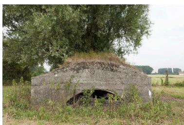
Casemate i, ouverture sud Phot. Jean-Marc Ramette IVR31_20145904937NUCA
