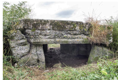
Elevation nord. Phot. Pierre Thibaut IVR32_20165900986NUCA
