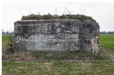
Elévation nord. Phot. Pierre Thibaut IVR31_20155900605NUCA
