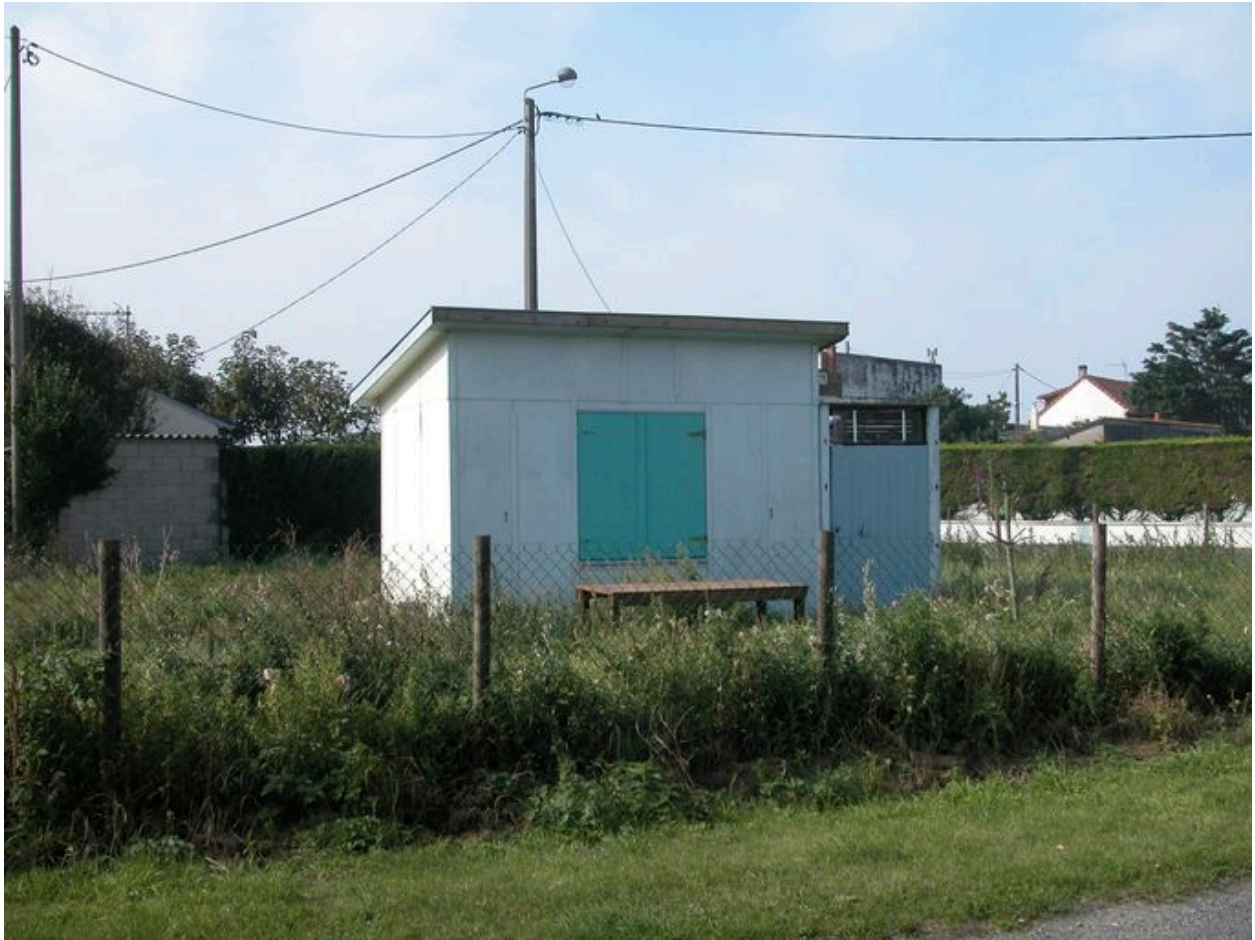
Bungalow, rue de Bougainville (1988 AY 175).
