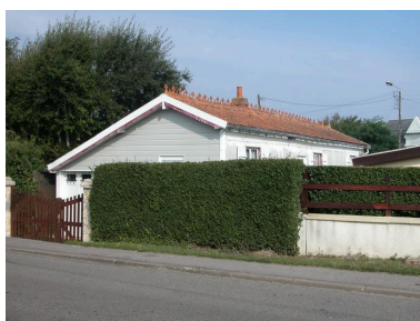
Maison, 8 rue Dumont-d'Urville (1988 AY 206). Phot. Elisabeth Justome IVR22_20058003103NUCA
