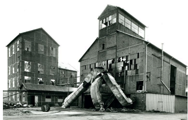
Chaufferie. Phot. Francis Dubuc IVR22_19908001158Z
