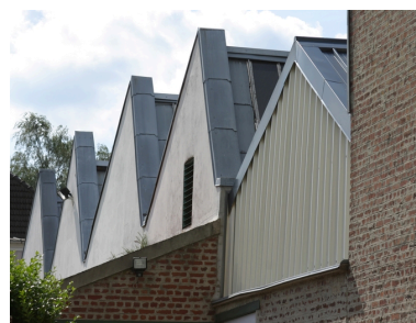
Les ateliers, couverts de sheds. Phot. Frédéric Pillet IVR22_20040200917NUCA
