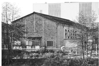
Magasin industriel, flanc est. Phot. Benoît Dufournier IVR22_19936002431Z
