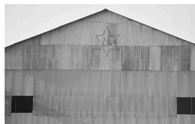
Magasin industriel : flanc est. Phot. Benoît Dufournier IVR22_19936002429Z
