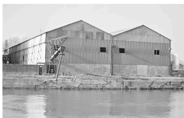
Magasins industriels : flanc est. Phot. Benoît Dufournier IVR22_19936002427Z
