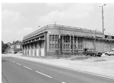
Stockage des pulpes. Phot. Francis Dubuc IVR22_19908000764Z
