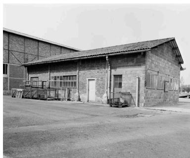
Atelier de réparation, angle nord est. Phot. Patrick Glotain IVR22_19936000457X
