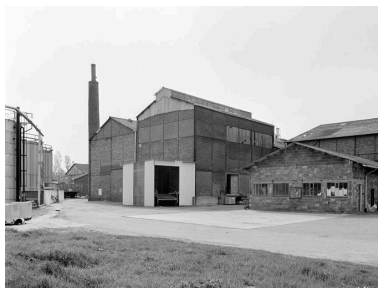
La chaufferie, pignon sud. Phot. Patrick Glotain IVR22_19936000458X
