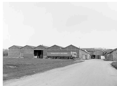
Ateliers de fabrication, pignons sud. Phot. Patrick Glotain IVR22_19936000452X
