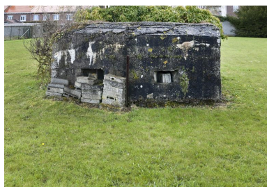
Elévation nord Phot. Jean-Marc Ramette IVR31_20145904292NUCA
