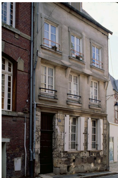
Elévation antérieure. Phot. Alain Nafilyan IVR22_19856001452ZA
