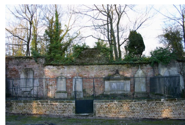
Enclos funéraire Morgan d'Epagny. Phot. Caroline Vincent IVR22_20098001589NUCA
