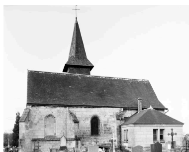
Élévation est. Phot. Jean-Michel Perrin IVR22_19846001404V
