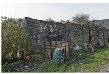
Elévation nord Phot. Jean-Marc Ramette IVR31_20145905517NUCA
