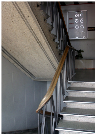
Services sociaux : escaliers. Phot. Frédéric Pillet IVR22_20040200834NUCA
