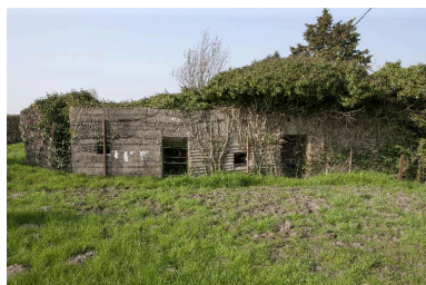
Elévation sud. Phot. Jean-Marc Ramette IVR31_20145905340NUCA
