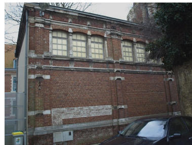
Vue partielle Phot. Bruno Decrock IVR31_20106202502NUCA
