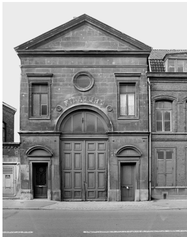
Bureaux, élévation. Phot. Olivier Marlard IVR31_19905900974X
