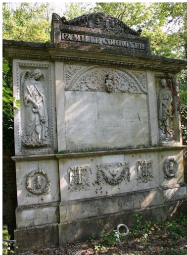
Tombeau-monument. Phot. Caroline Vincent IVR22_20068001439NUCA
